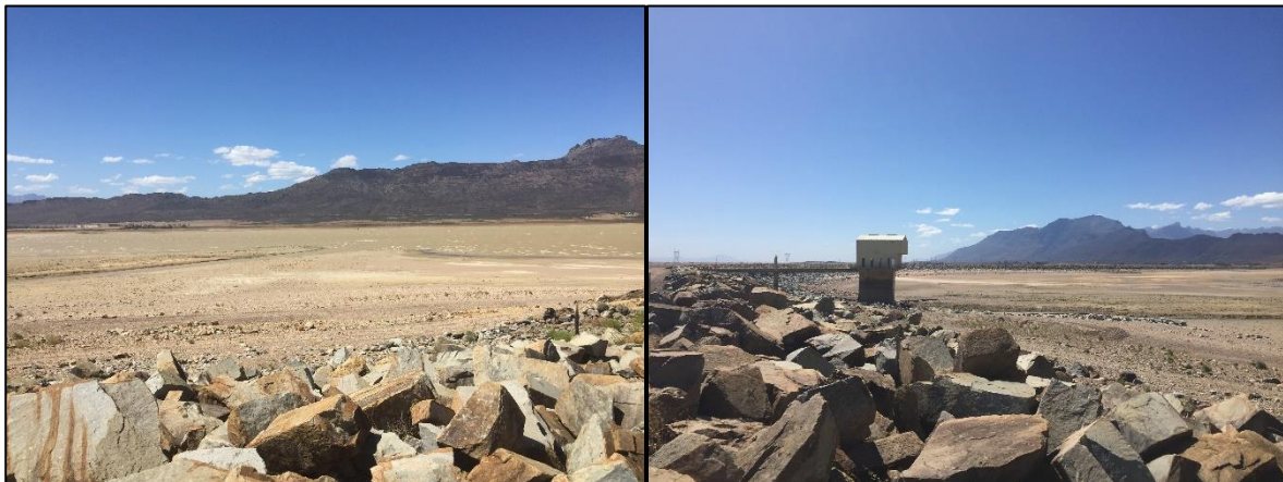
Figure 23: Images of the low water levels of the Voëlvlei Dam
